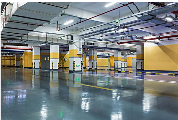
Fig.3 Underground parking lot
