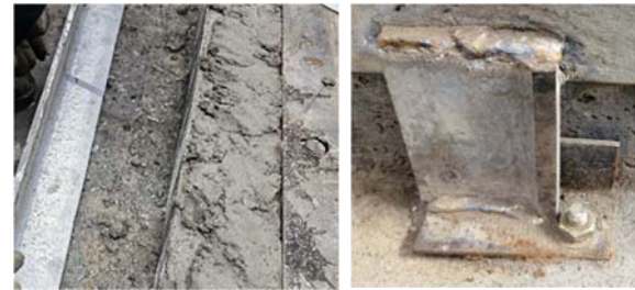
FIG. 4 SCHEMATIC DIAGRAM OF CONCRETE FOUNDATION POURING AND ANGLE STEEL FIXATION
